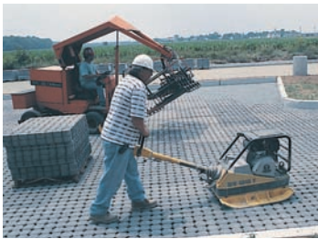
Pavers are delivered ready to place, joints filled, compacted and then are ready for traffic.
