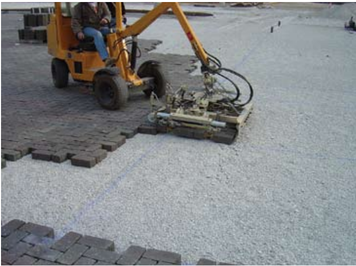
Figure 4. Many PICP projects are mechanically installed thereby decreasing construction time and labor costs because many pavers are placed at the same time.
