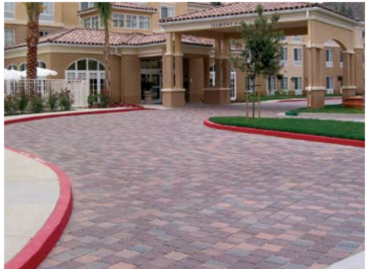
Figure 5. PICP color and texture compliments the architecture of a Hilton Garden Inn in Calabasas, California while communicating the sustainable nature of the site.
