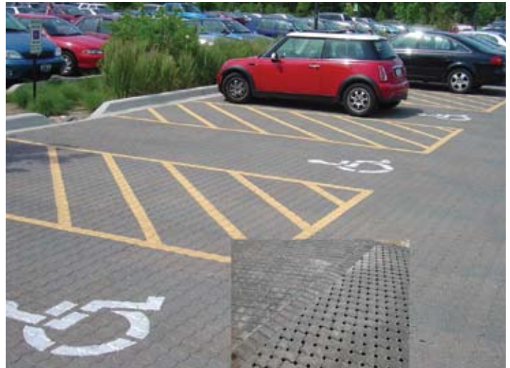
Figure 7. PICP combined with solid interlocking concrete pavers accommodates accessible parking and pedestrian areas.
