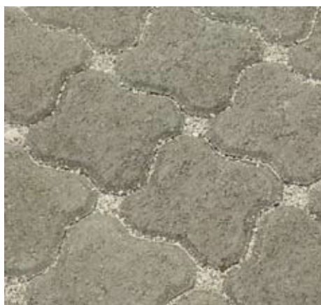
Figure 3. Left to right: After excavation, PICP construction begins with placing and compacting an open-graded subbase and base as shown in the first two photos. The next photo shows mechanical installation of the concrete pavers on a screeded bedding layer of small aggregate. The rightmost photo illustrates small aggregate in the openings and joints that enable high surface infiltration. The pavers and aggregate are compacted to create an interlocking pavement.
